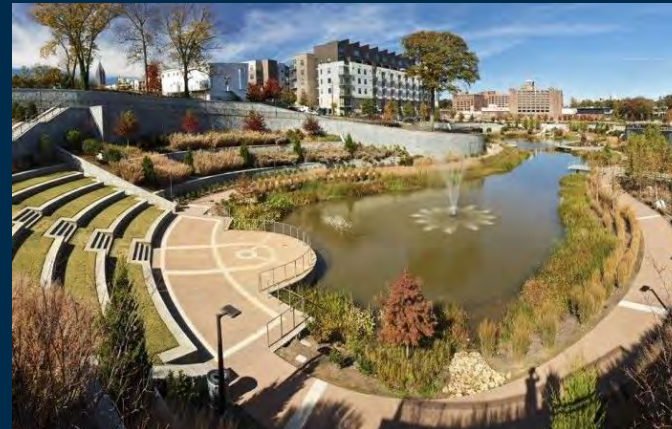
Regional Detention Pond
